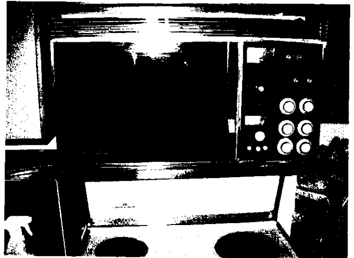
Unit #2 - Kitchen—Exhaust Vent Fan —The exhaust vent fan above the range was not operating at the time of inspection. Recommend repairing or replacing the exhaust vent fan.
