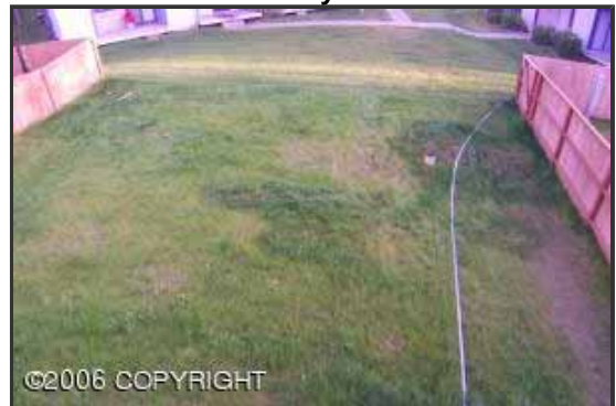
Fence along back would enclose. Drain line for sump pump shows
